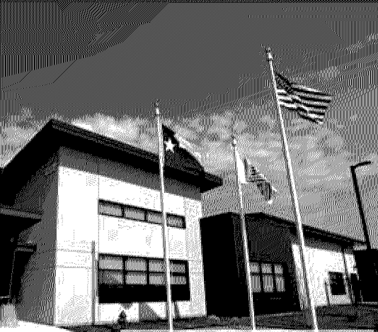
Leonard Water Treatment Plant
